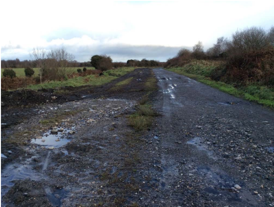
Plate 61: Continuation of proposed (and existing) access road looking northeast.
