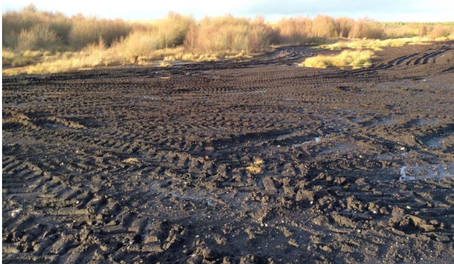
Plate 87: Proposed road between construction compound and T17 looking north.
