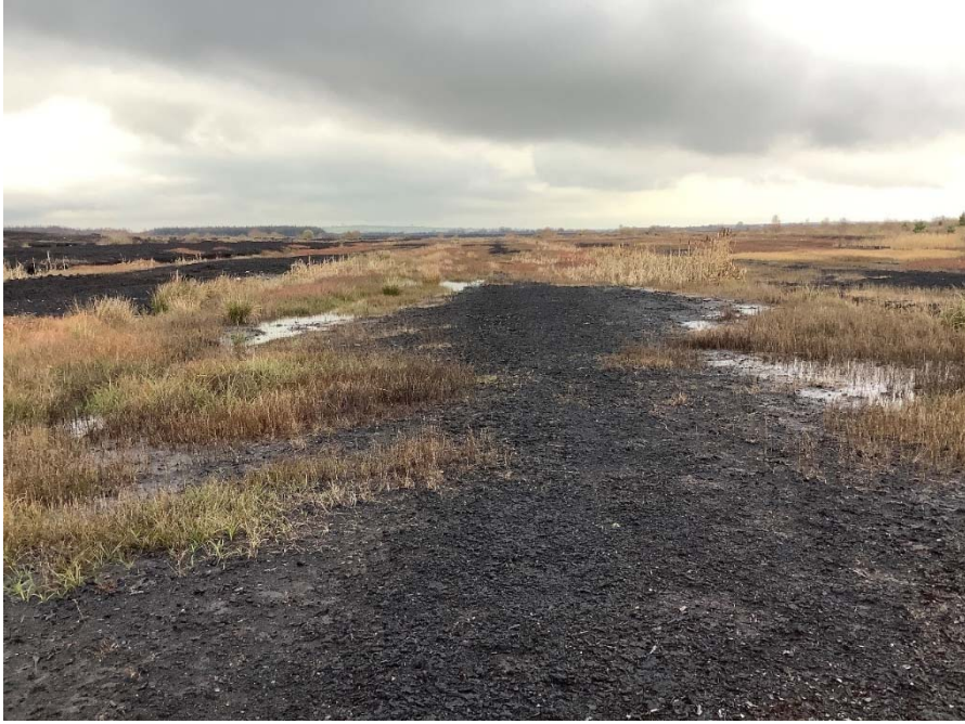
Plate 24: General vicinity of Turbine 6 and hardstand looking northeast.
