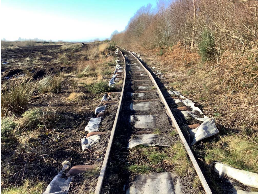
Plate 144: Trail looking west along industrial railway tracks.
