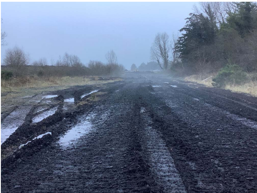
Plate 59: Proposed construction access track commencing at N62 looking east.
