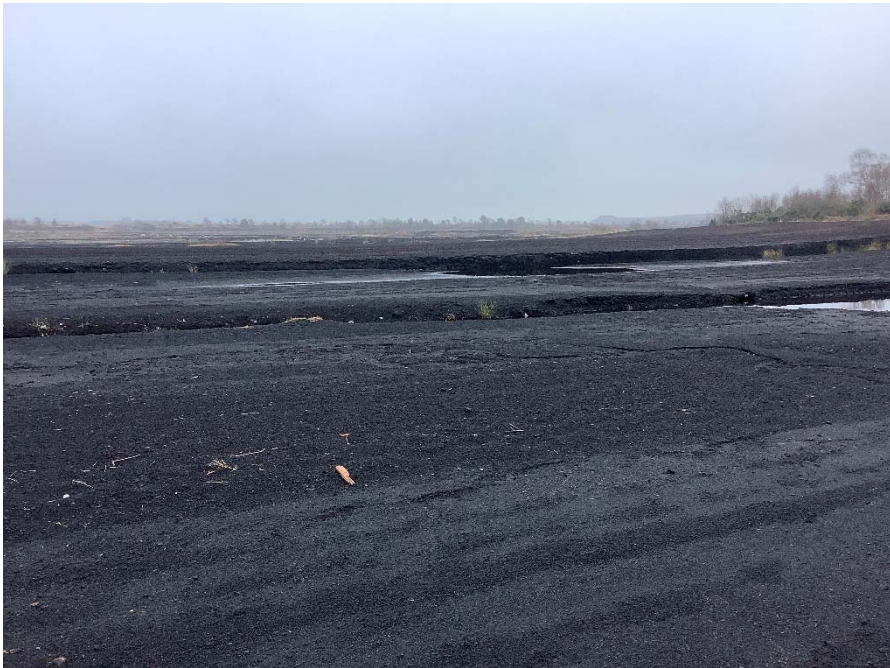
Plate 105: View towards eastern end of construction compound looking east.
