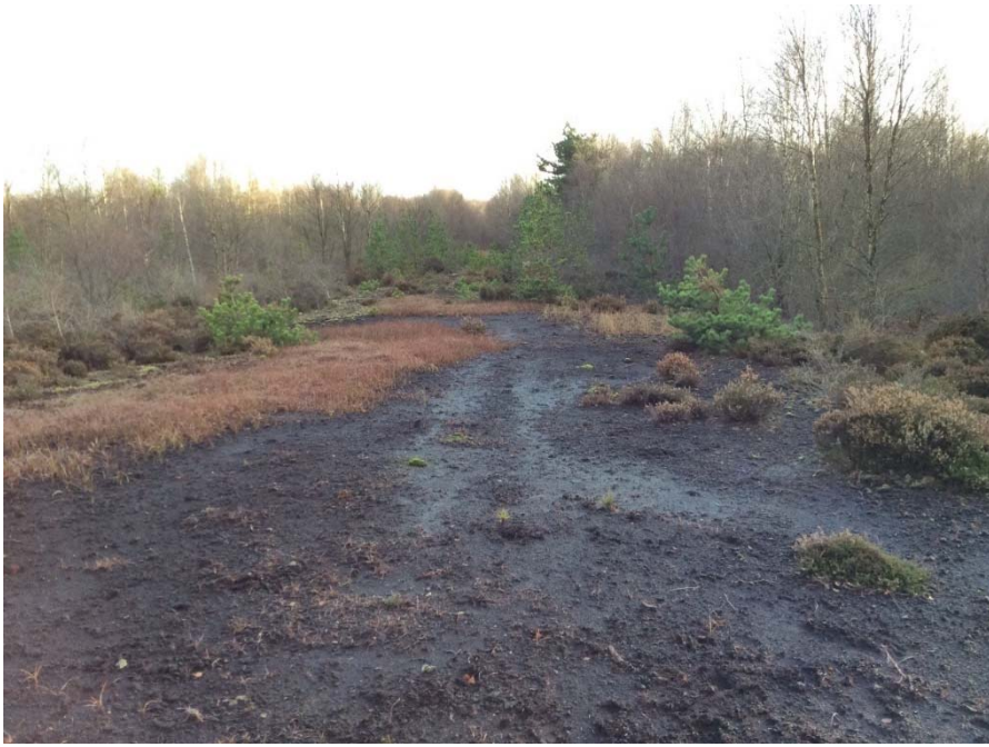
Plate 84: Construction compound looking south.
