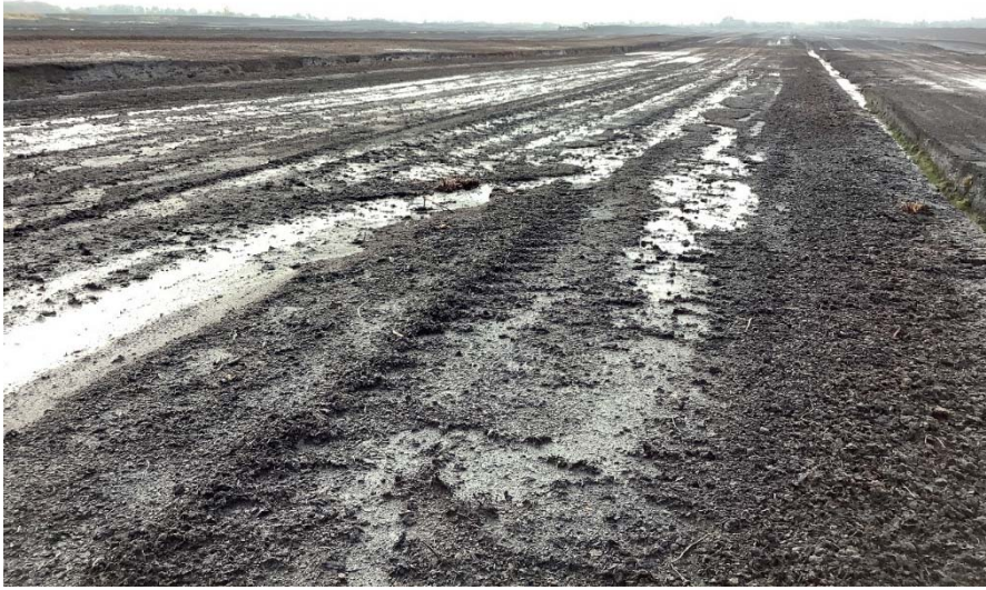
Plate 18: Area of T5 turbine base looking south.
