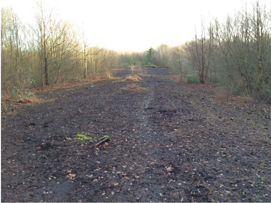
Plate 86: Centre of construction compound looking south.
