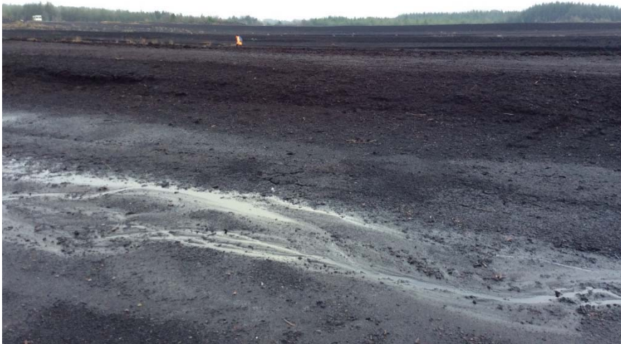
Plate 11: T3 hardstand (western extent) looking east.
