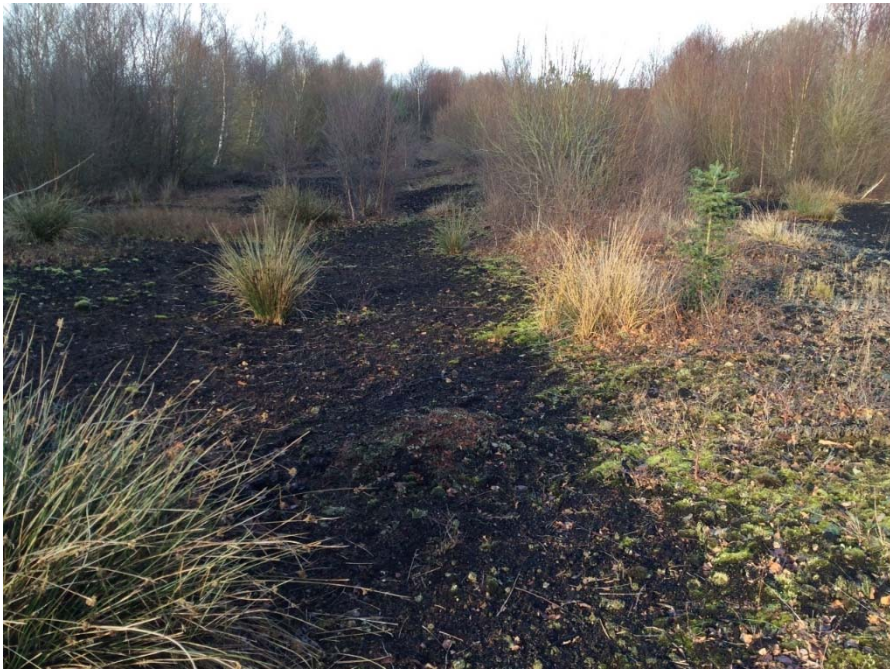
Plate 101: Hardstand for T21 looking north.
