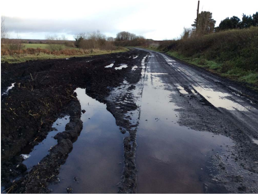
Plate 60: Proposed access to the Drinagh section of the windfarm looking east.
