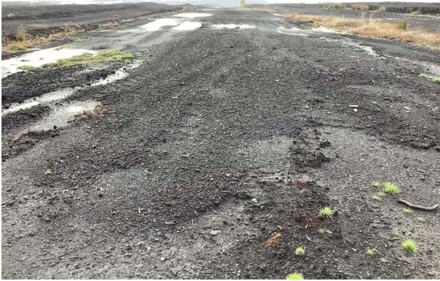
Plate 10: T3 turbine base looking west.
