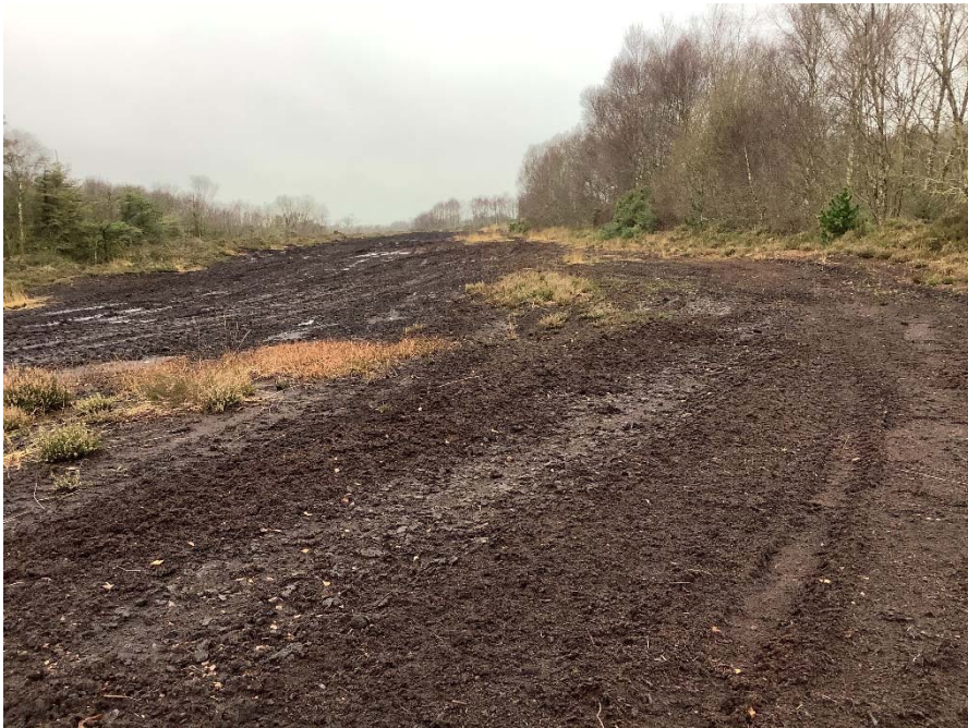
Plate 121: Proposed road looking west before it turns south to T21.
