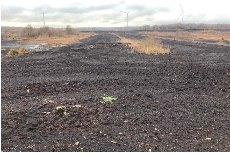
Plate 34: Hardstand for T9 looking southwest. Meenwaun turbines in background.
