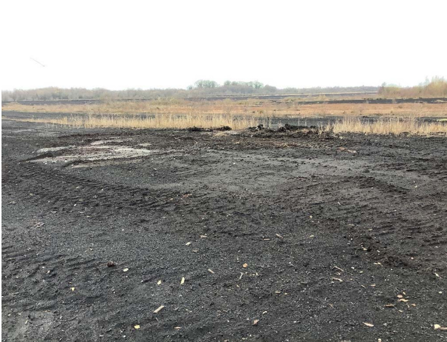
Plate 35: T9 turbine base looking southwest.
