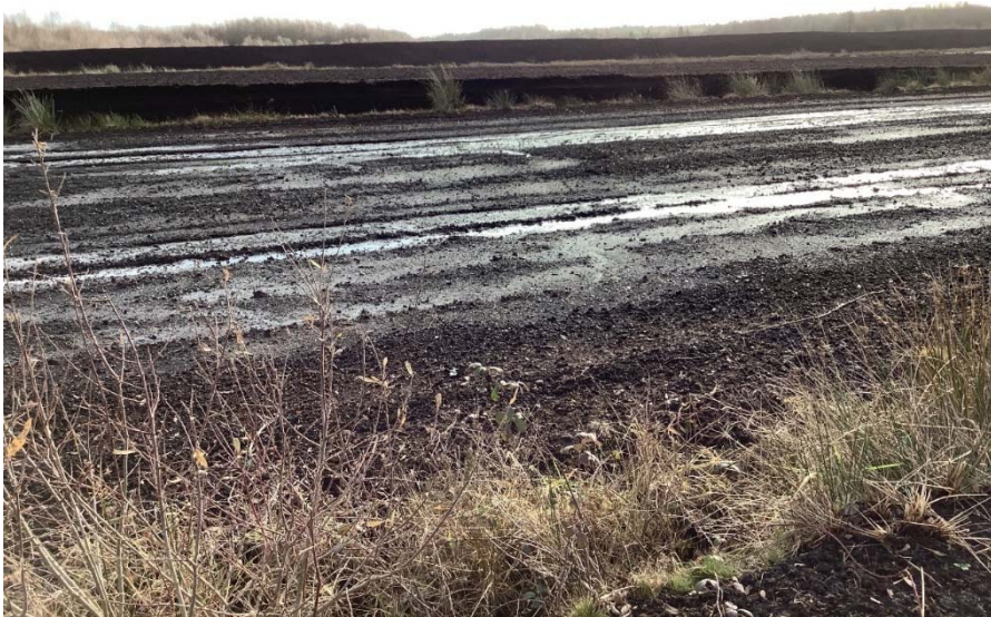
Plate 43: Continuation of proposed road into T11 looking southeast.
