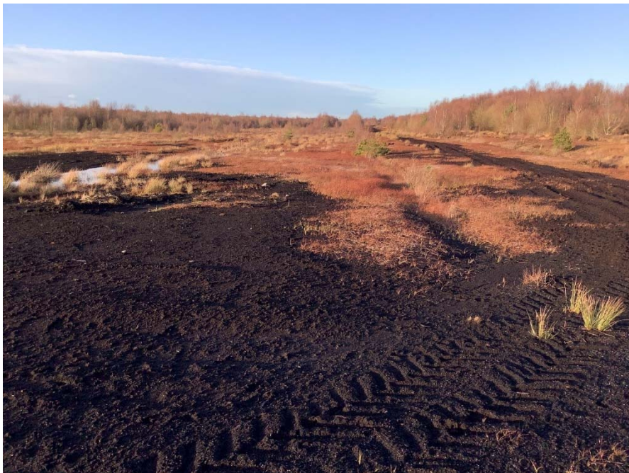
Plate 83: Proposed road from T16 to proposed construction compound and T17 further to the north, looking north.
