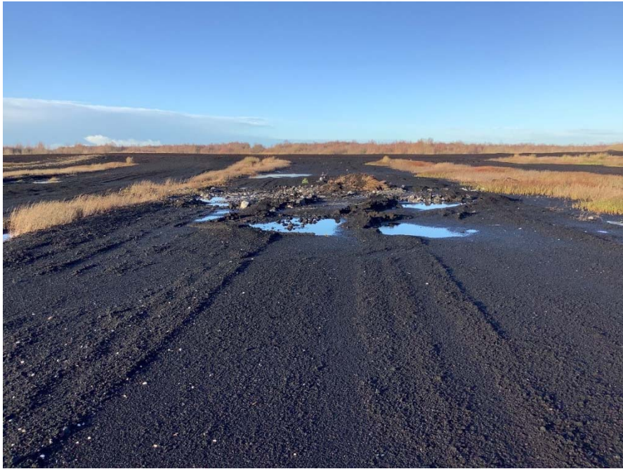
Plate 78: T16 turbine base looking north (excavated trial pit within base).
