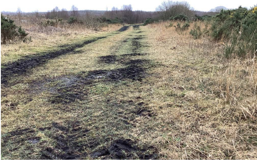
Plate 118: Continuation of road looking south/southwest.
