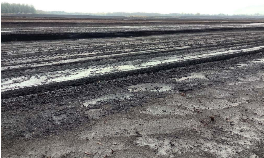
Plate 17: Hardstand for T5 looking south.
